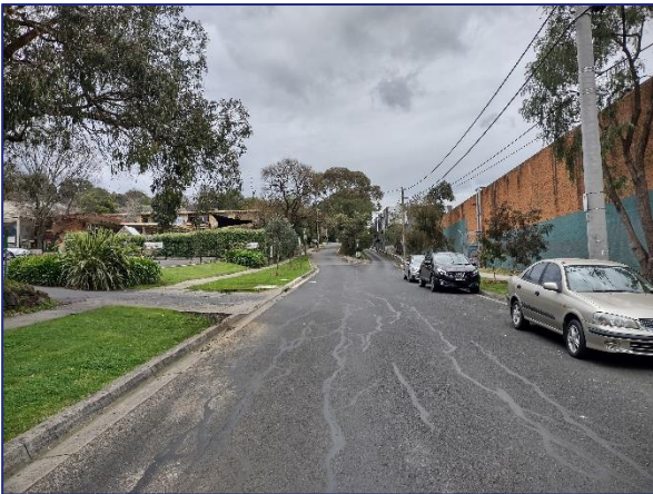
Figure 13: Toorak Avenue – view north
