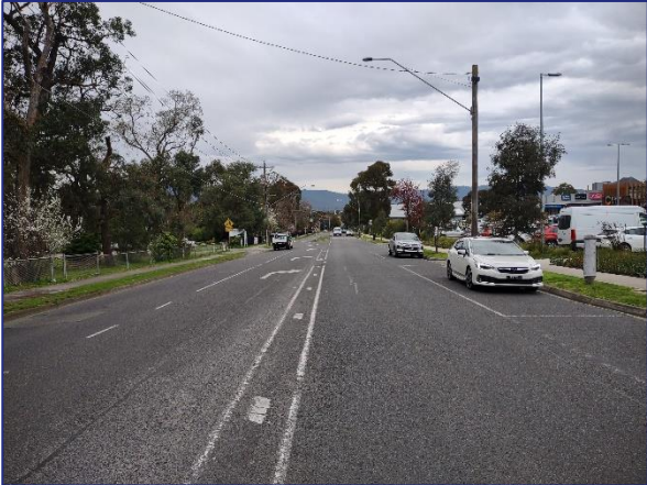
Figure 10: Kent Avenue – view south
