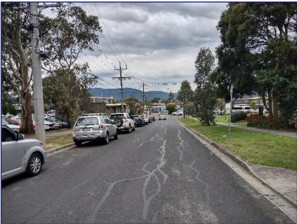
Figure 14: Toorak Avenue – view south
