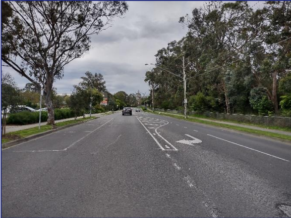
Figure 9: Kent Avenue – view north
