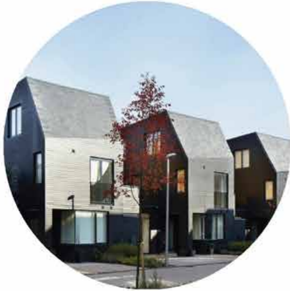
NEW TOWNHOUSES TO TOORAK AVENUE
