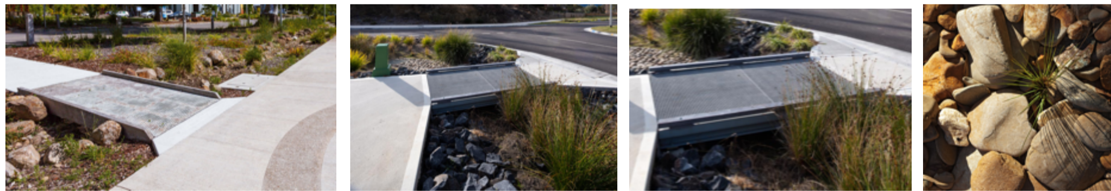
bridges and treatment across vegetated swales
