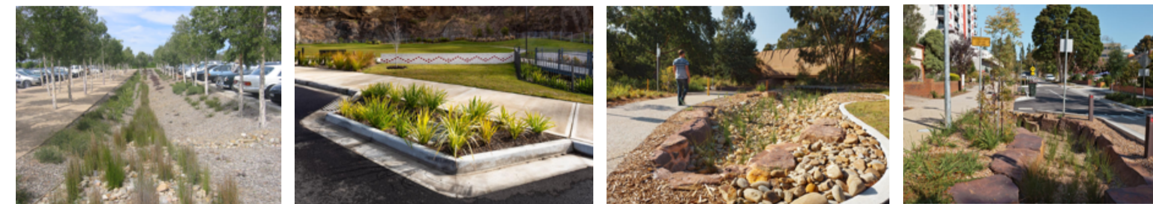
water sensitive urban design to integrate proposed carpark upgrade within the landscape characteristics of the site, treating swales with ephemeral indigenous planting palette and extending soil moisture and ground water
