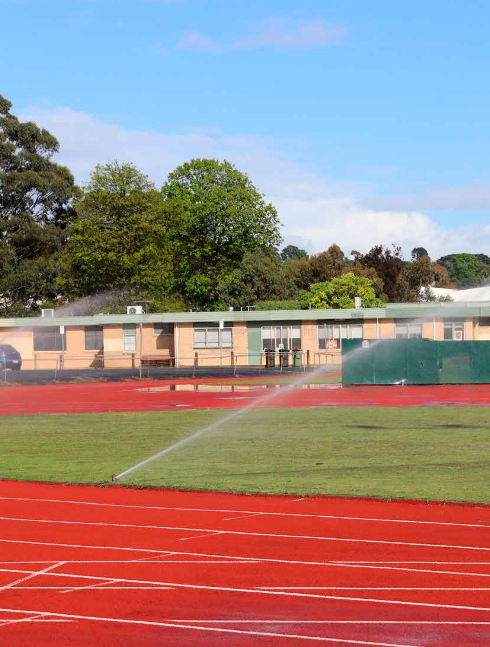
Stormwater harvesting at Croydon Town Park
